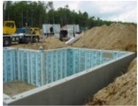
Fig no: 103 Pre cast Concrete Foundation
