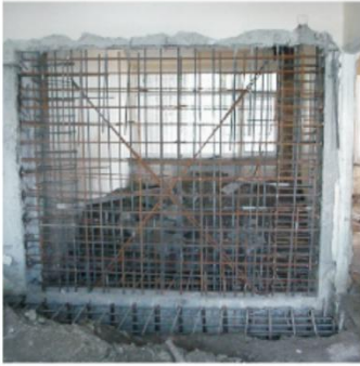
Fig no: 76 Additional shear wall
